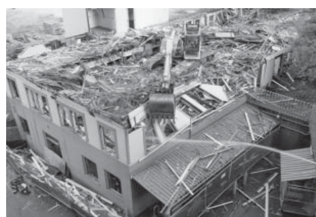
Down comes the first-floor wall of Johnson Annex.
